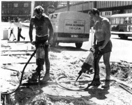
The 1970's. first TEX series with noise suppressing muffler bags .... and with polyurethane jacket cutting noise by 50%, compared with a standard breaker.
