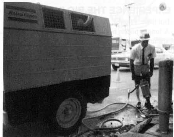
The 1970's. first TEX series with noise suppressing muffler bags .... and with polyurethane jacket cutting noise by 50%, compared with a standard breaker.
